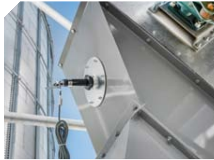
Plug switch option in head discharge eliminates potential overload concerns.
